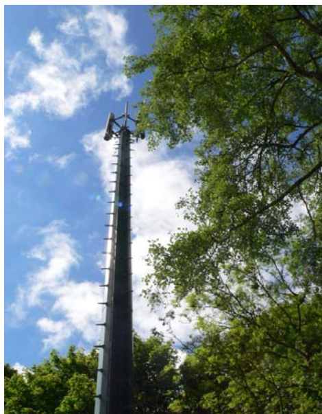
Example of mast screened by trees
