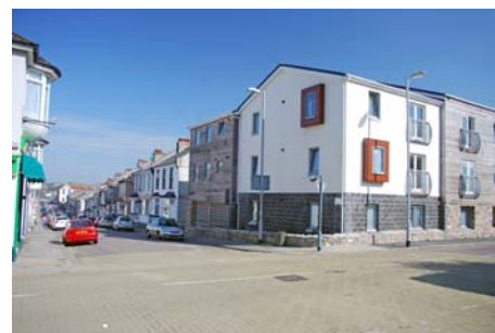
Flats built to Lifetime Homes Standard
